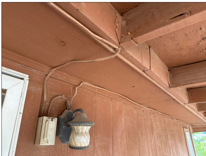
recommend protecting electrical cables at exterior
