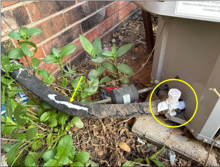
unit froze up upon operation; recommend further evaluation
