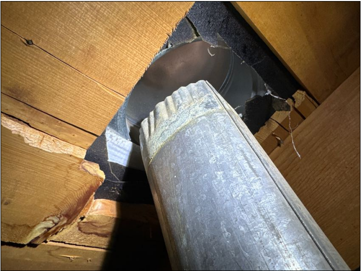
original dryer vent not properly sealed to roof vent
