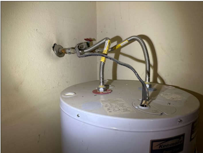
no proper service disconnect
