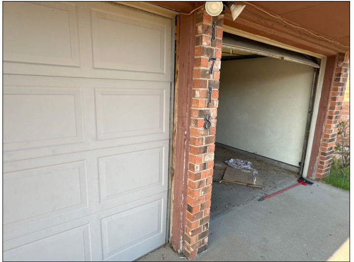
missing weatherstripping
