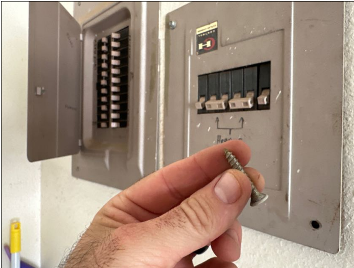
sharped-tipped screws not approved
