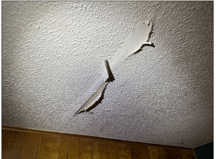
previous water damage example
