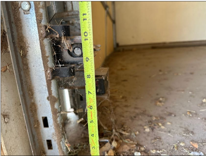
reverse eyes installed higher than max 6"
