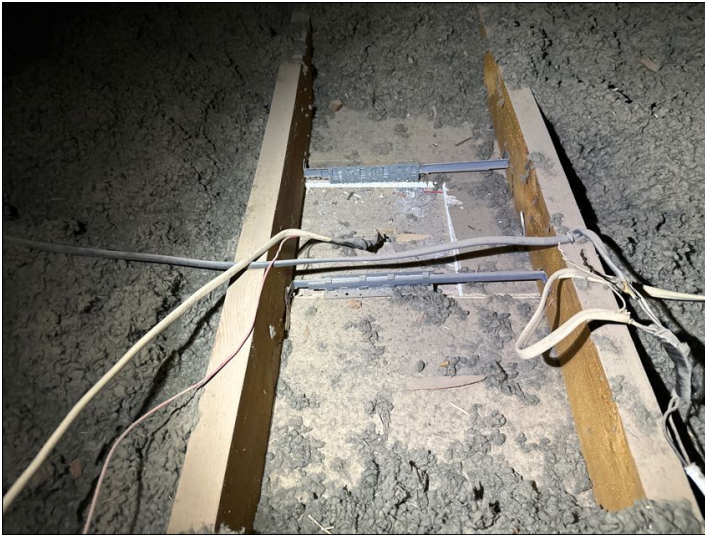
insulation missing/low example
