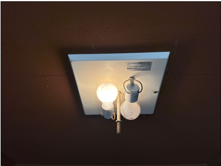
missing fixture cover - front porch
