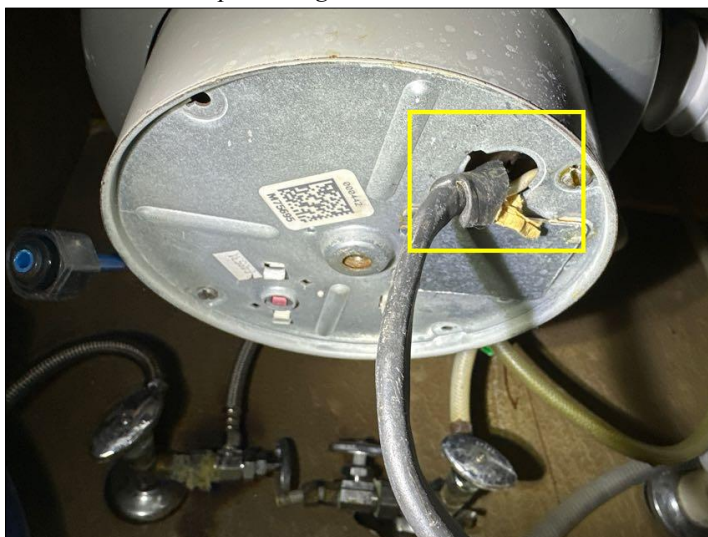
example of missing cable clamp
