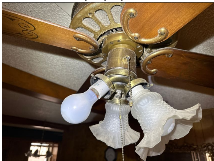
missing fixture cover
