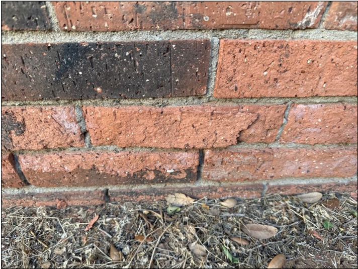
brick spalling example
