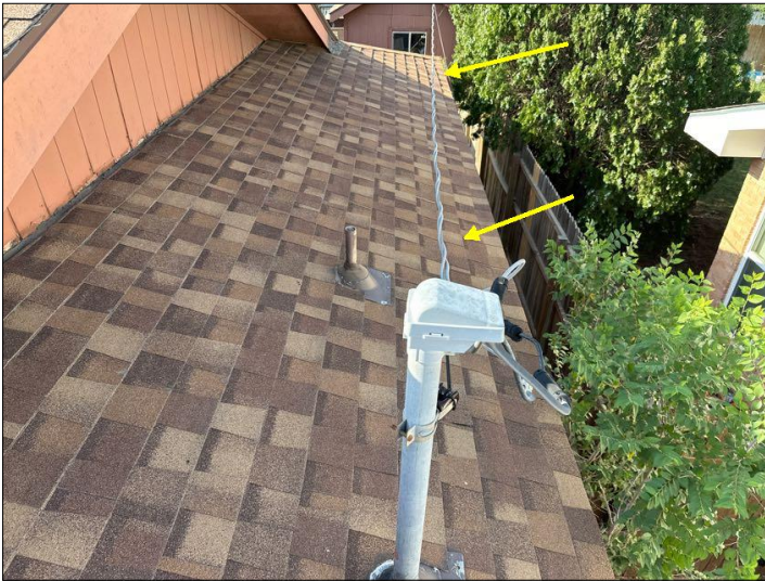
insufficient roof clearance per modern standards
