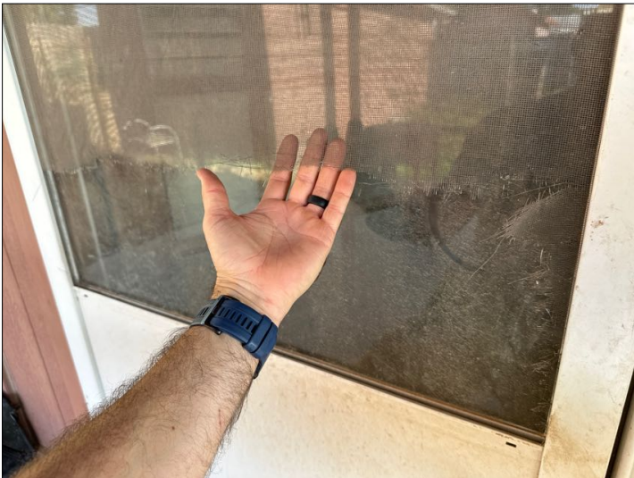
damaged storm door screening
