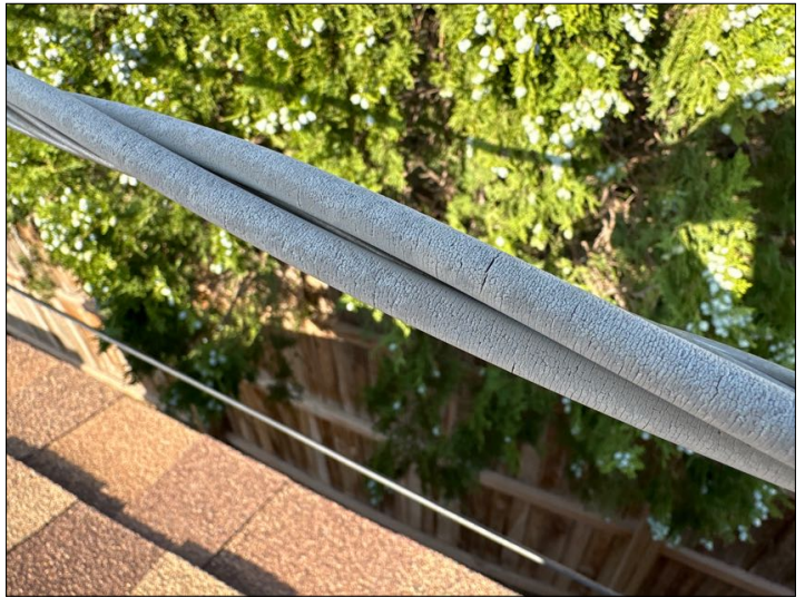
cracks/wear on sheathing of overhead cables
