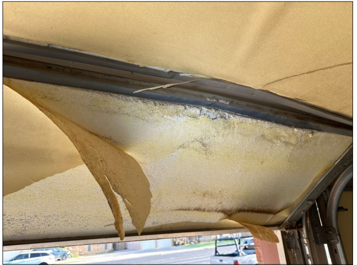
garage door damaged/bending
