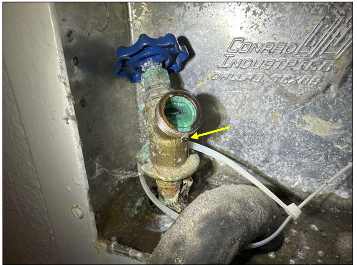
dripping/slow leak from laundry hose bibb connections
