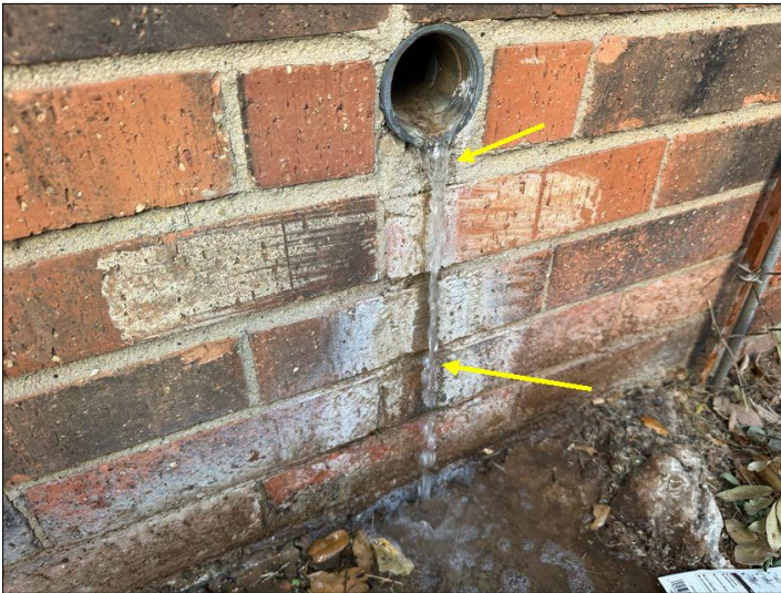
kitchen sink drains out cleanout due to blockage downstream
