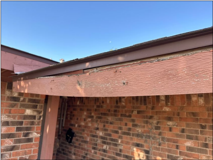
water damaged fascia example
