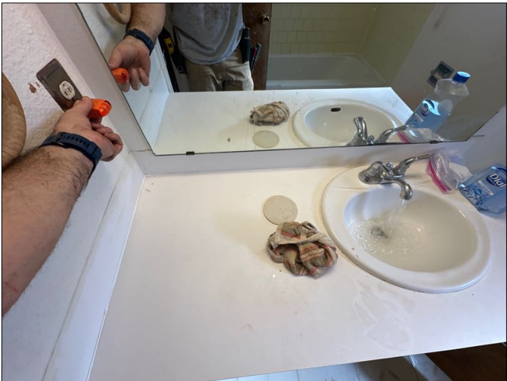
recommend GFCI in bathroom(s)
