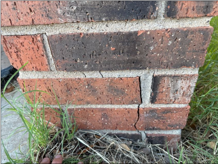
thermal/expansion crack example
