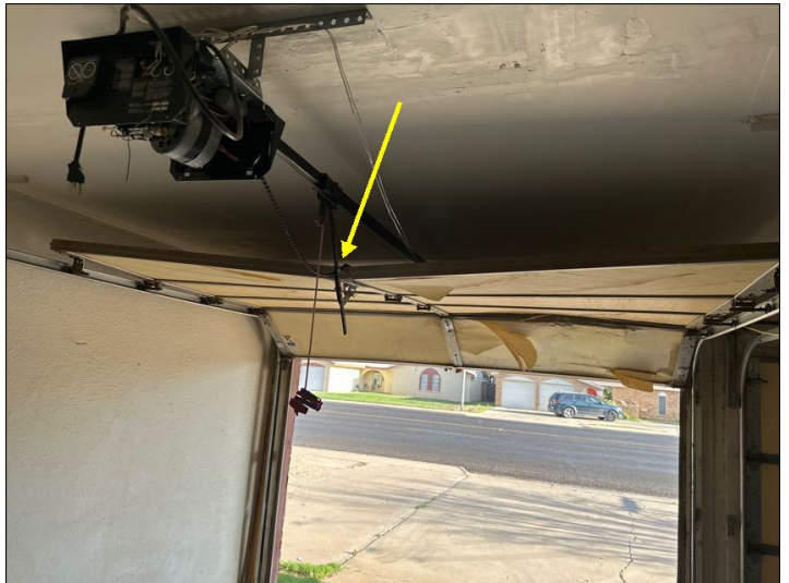
garage door damaged/bending
