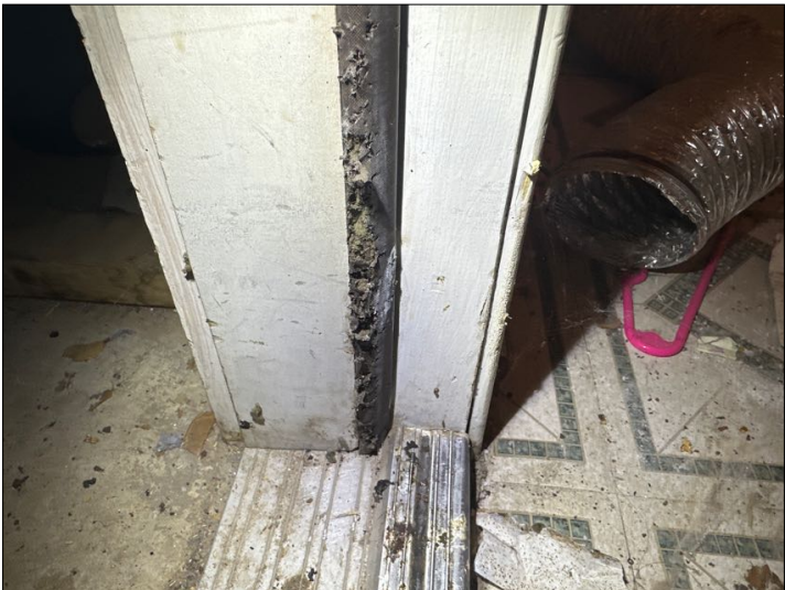
weatherstrip damaged/missing
