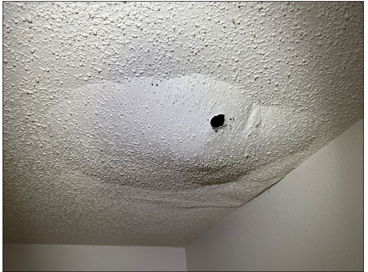
previous water damage example
