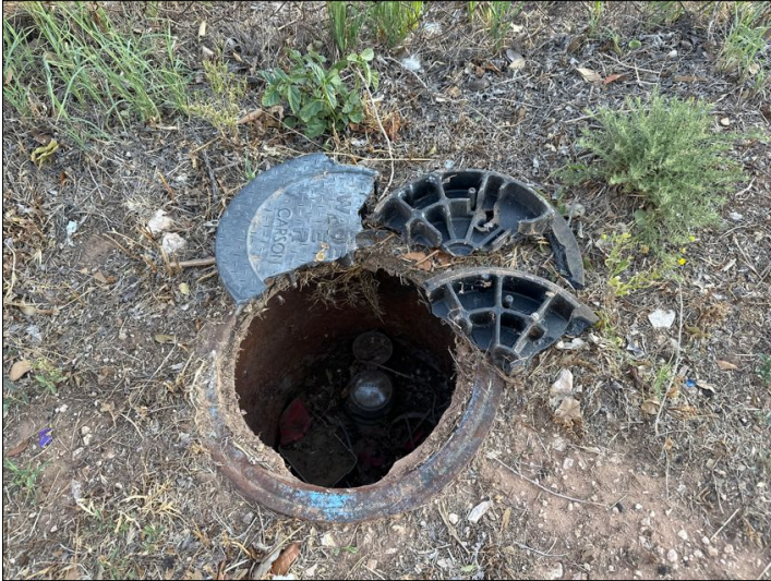
water meter cover broken
