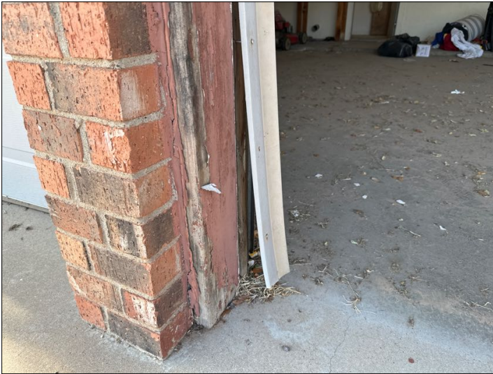
missing/damaged weatherstrip
