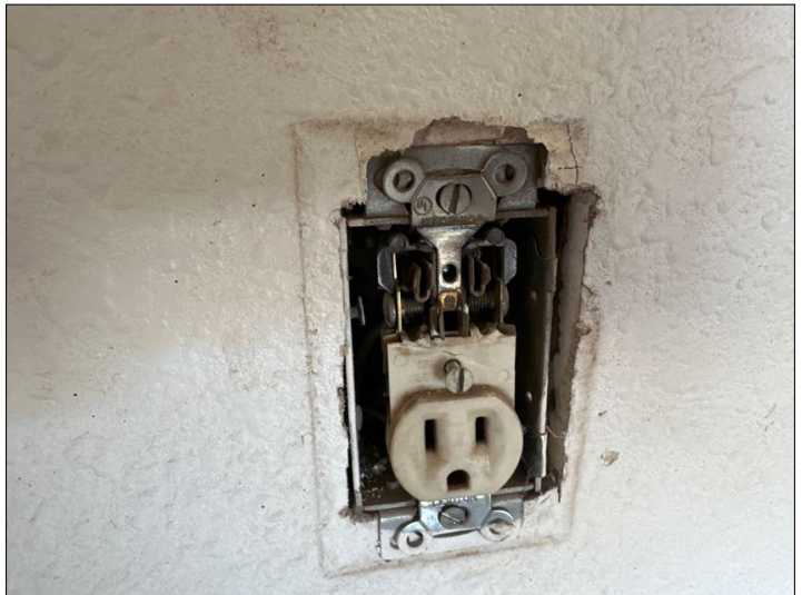
replace damaged receptacle in garage
