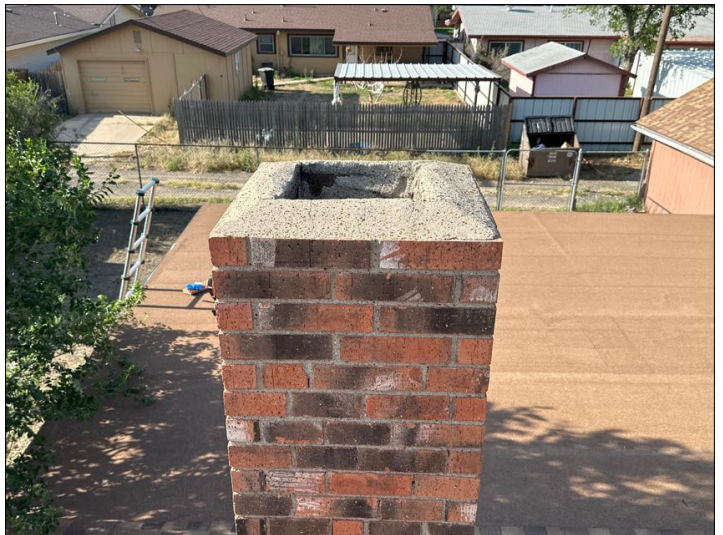
recommend spark arrestor/rain cap
