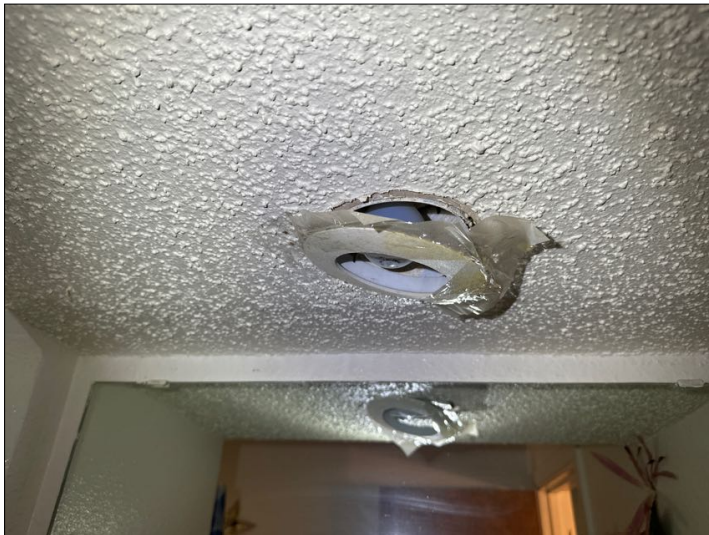
loose light fixture cover
