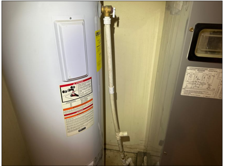
TPR piped out with PVC
