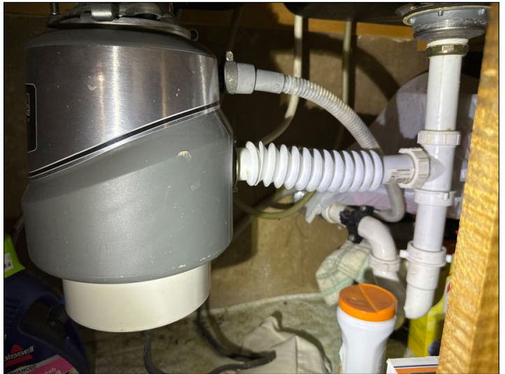
flex/corrugated drain line at kitchen sink
