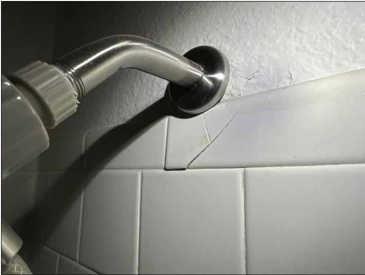
cracked tile example
