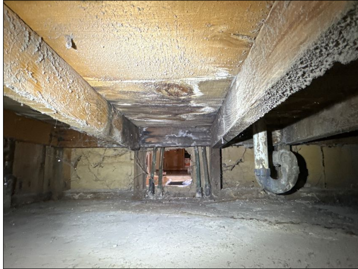
previous water damage in return air chase
