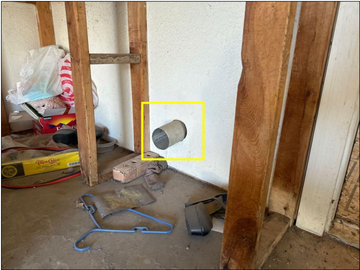
dryer vent terminates into garage; extend to exterior
