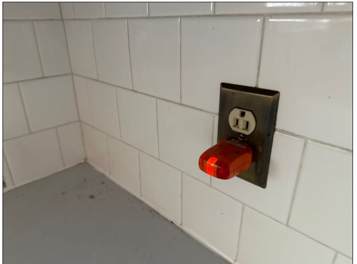
open ground receptacle in kitchen
