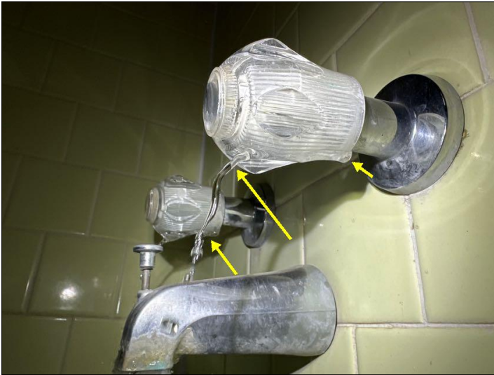
leaking shower valves - guest bathroom
