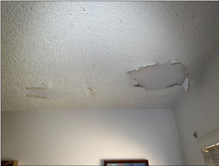
previous water damage example
