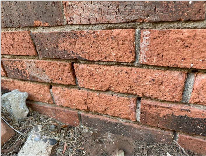
brick spalling example
