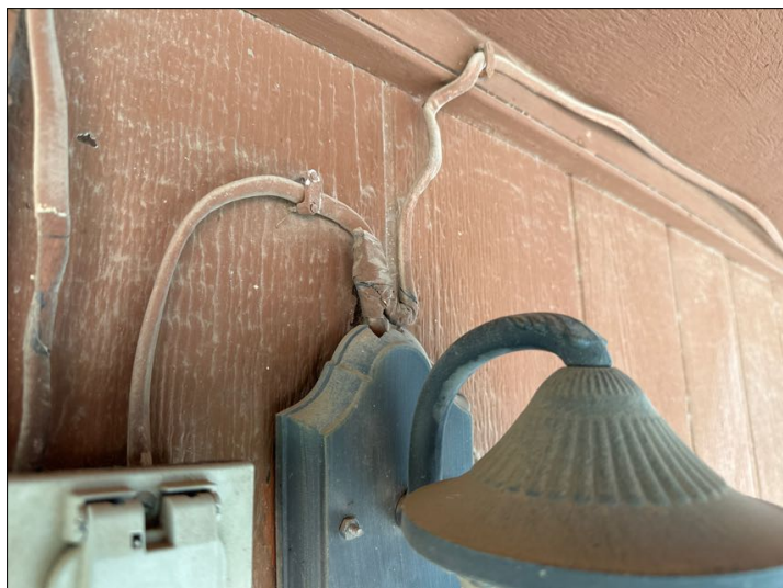
repair open splice
