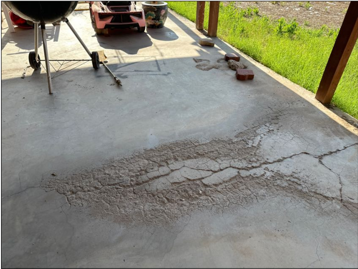
general wear/spalling example
